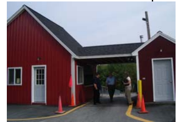
Chester Transfer Station: Scales
