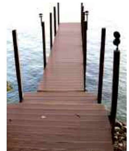
Verdura™ Decking at the Lake
